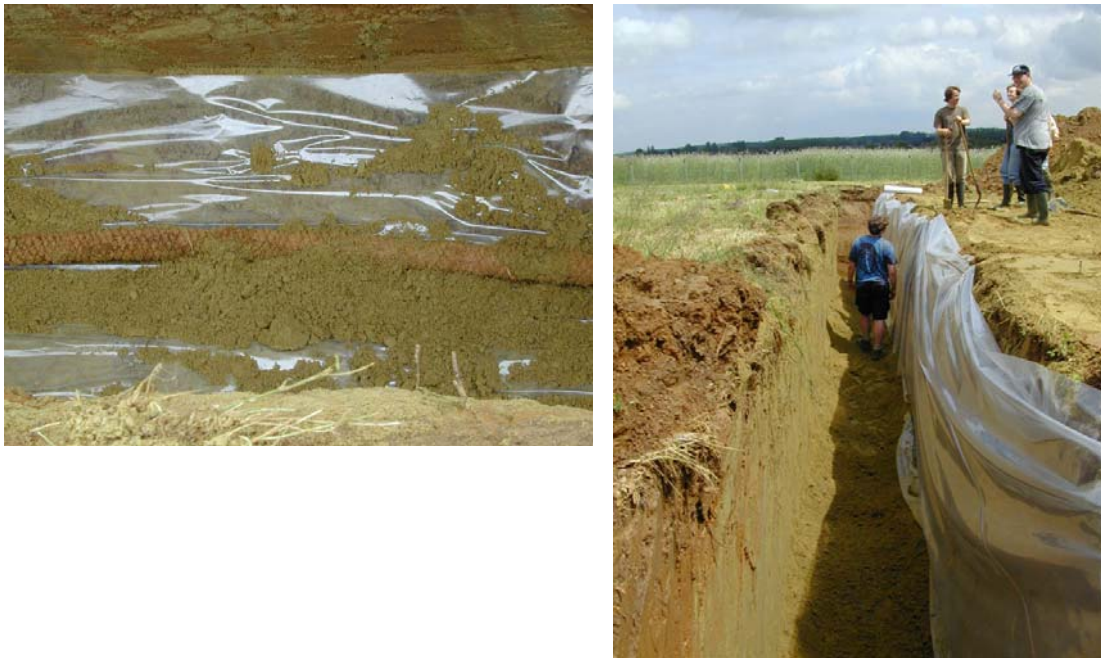
Figure 2.8 Installing drains in trench at bottom of experimental plot
