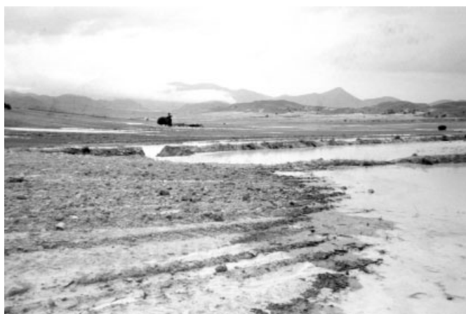
Figure 11. Runoff at highest level of scale on 29 September 1997, in the upper Cañada de Hermosa valley bottom, the upper source area of the Campo de Panes catchment. All water-retention dams are breached by continuous accumulation of overland flow
